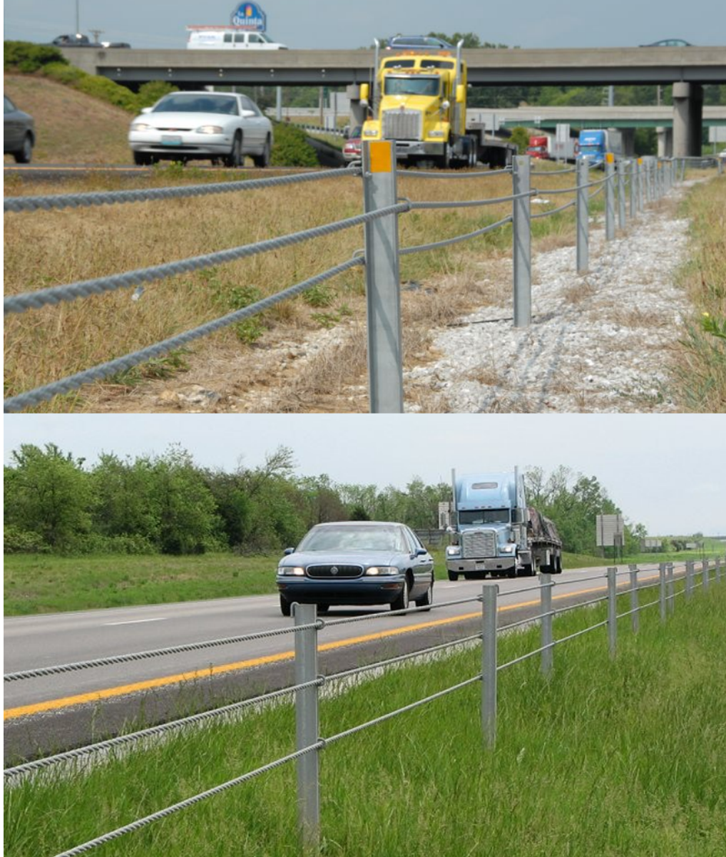
Figure 1: Low-Tension Cable Barrier (top); High-Tension Cable Barrier (bottom)
